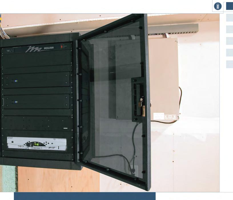
dust, and other hazards, and many styles have hinged center sections to provide enhanced rear access to equipment and wiring.
